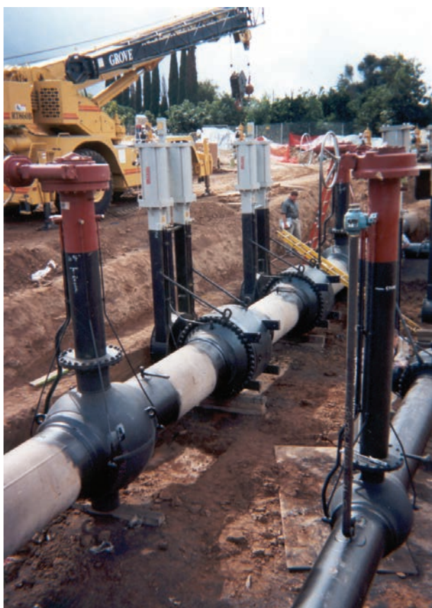
Figure 1 – Installation of Becker Below Ground Ball Valve Regulator
