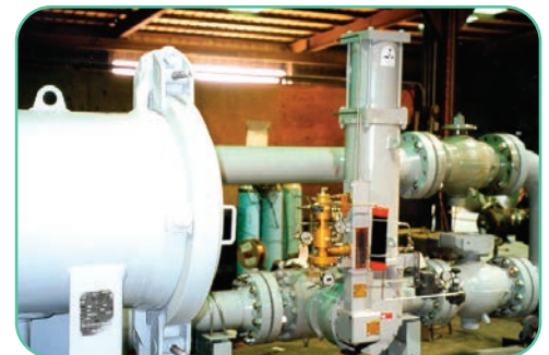
Figure 14 – Becker RPSR Actuators are ideal for Surge Control/Recycle Valves
