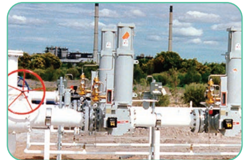
Figure 13 – Becker RPSR Actuated Control Valves in Power Plant
